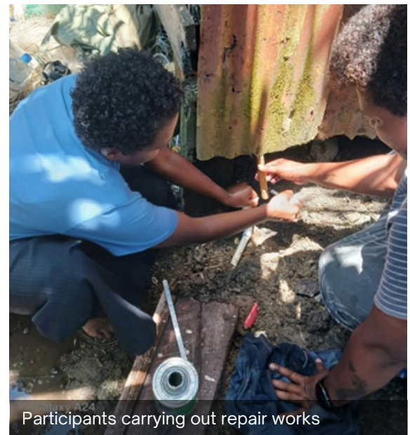
Participants carrying out repair works
