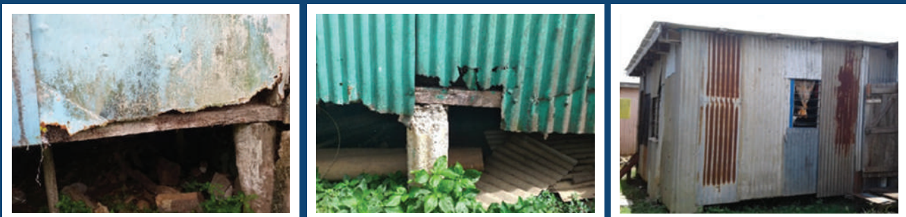
State of sheet metal walls over time
