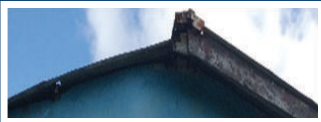
Missing barge boards exposes the purlins to harsh weather conditions.
