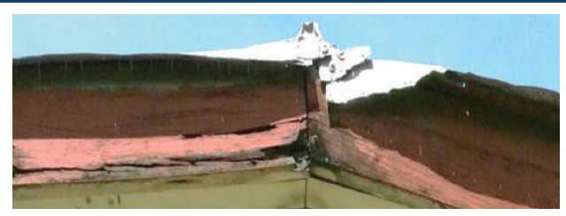
Rotten barge boards
