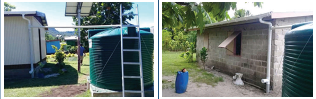
Typical rainwater harvesting system
