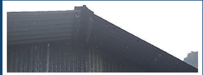
Missing barge boards exposes the purlins to harsh weather conditions.
