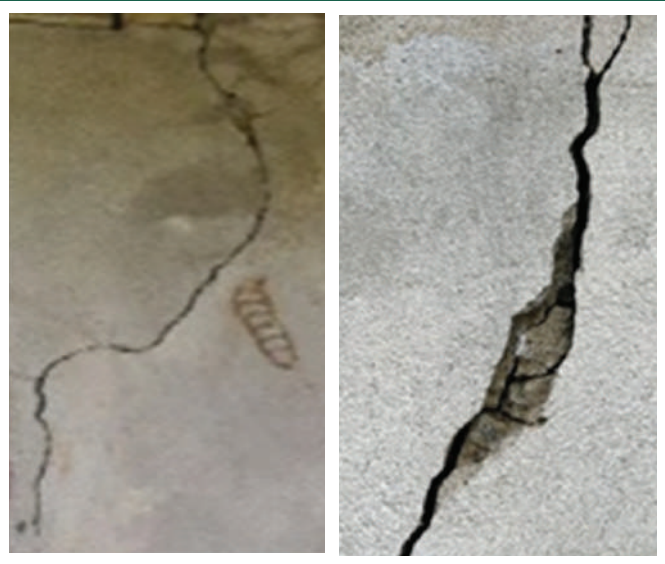
Hairline cracks
