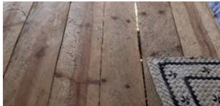
images of rotten and loose floorboards and floorboards with many knots
