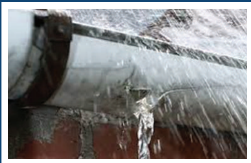
! Leaking gutters
