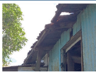
Corroded corrugated roofing iron
