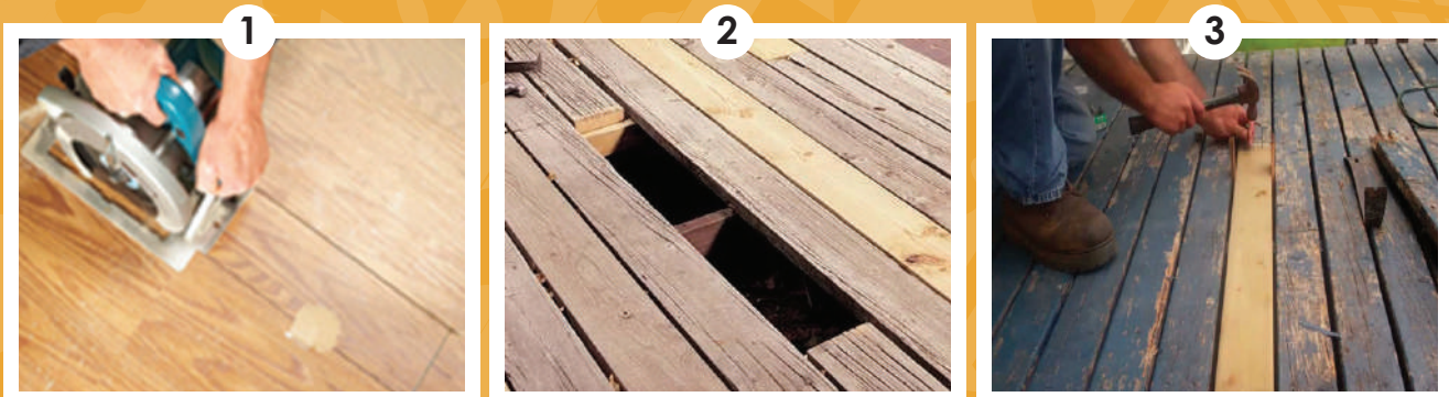
1 Cut out rotten floor
