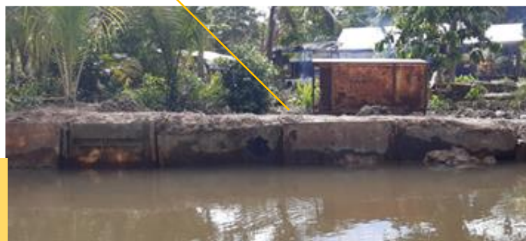
Old fridges used on river channel to minimize bank
