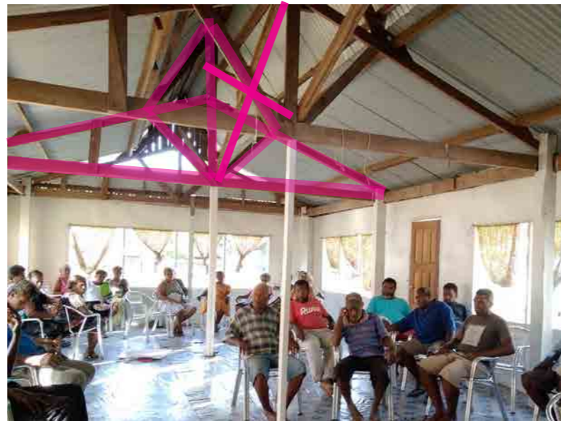
Figure 52: Dutch Gable roof truss for corrugated galvanized steel roofing at a community hall Location: Jabros settlement (Photo credit: John Clemo)
