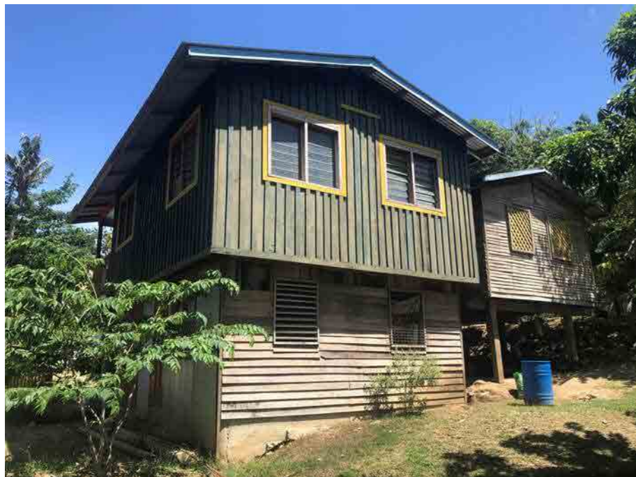
Figure 62: Housing recovery for some: houses with enclosed lower floor for accessibility. Location: Aekafo-Feraladoa settlement (Photo credit: John Clemo)
