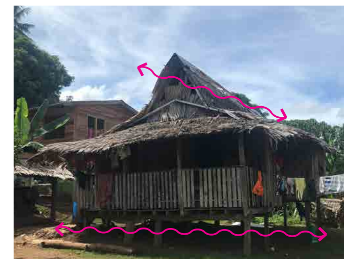
Figure 12: Photo of a traditional house with Dutch gable roof, lower leaf roof and upper steep roof. Location: Jabros settlement (Photo credit: John Clemo)
