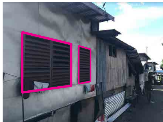
Figure 56: Openable timber louvre shutters on windows for wind and rain protection. Location: Ontong Java settlement (Photo credit: John Clemo)
