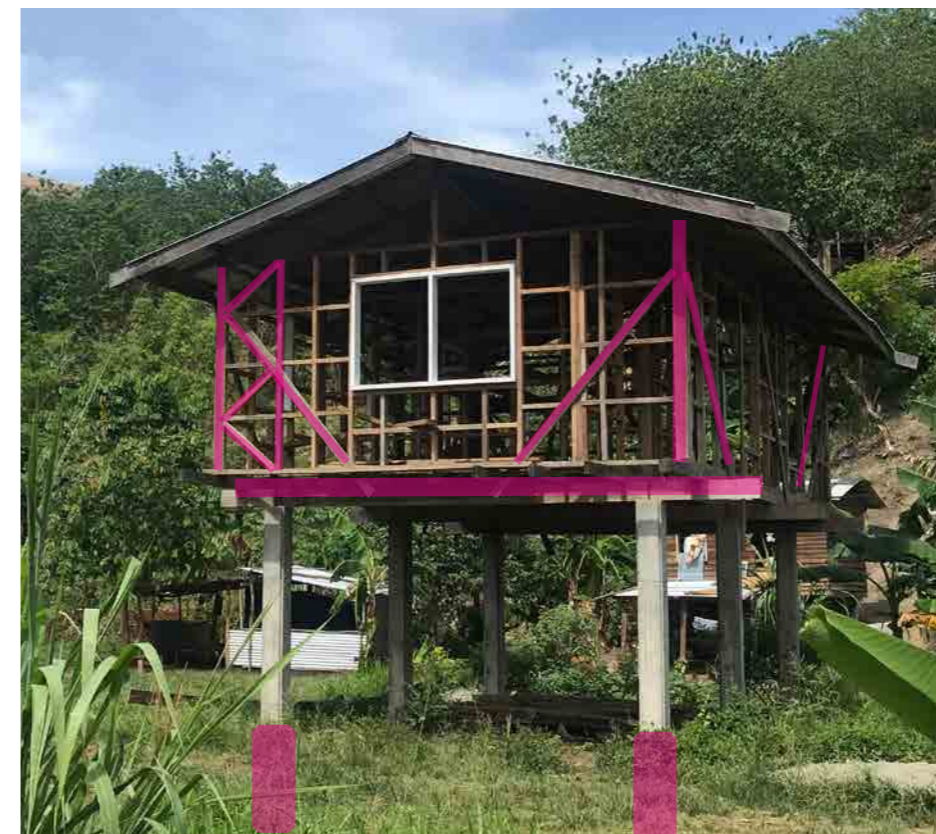
Figure 59: Incremental house with timber framing on reinforced concrete posts. Location: Jabros settlement (Photo credit: John Clemo)
