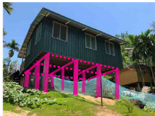
Figure 13: Photo of a 'strong' house built by Kwara'ae man; dotted line shows improvement opportunities. Location: Wind Valley settlement (Photo credit: John Clemo)
