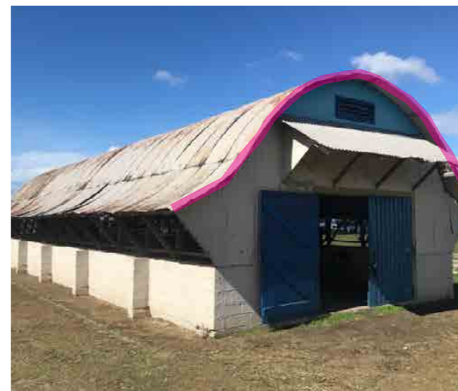
Figure 55: (Left) Photo of round roofed building, which has withstood a number of cyclones. Location: Solomon Islands National University Campus (Photo credit: John Clemo)
