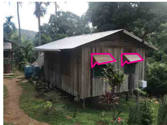
Figure 57: Fixed rain-guards in a semi-traditional house. Location: Aekafo-Feraladoa settlement (Photo credit: John Clemo)
