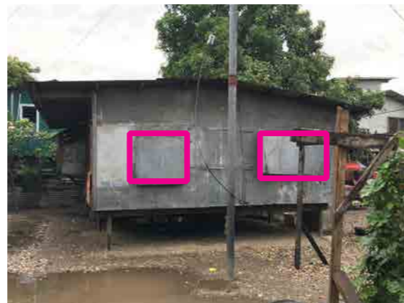
Figure 58: Openable copper sheet shutters on windows for wind and protect on rain. Location: Ontong Java settlement (Photo credit: John Clemo)
