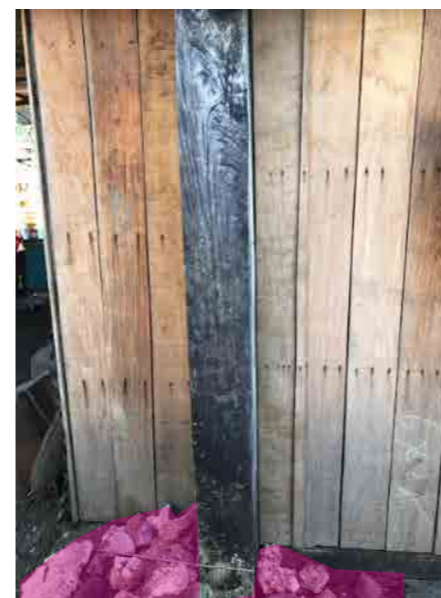
Figure 37: Photo of a house with crushed coral footing and timber post, which is painted with tar to protect from white ants and decay. Coral rocks are also added around the bottom of the wooden post to provide a bit of buffer and protection from waves. Location: Ontong Java settlement (Photo credit: John Clemo)
