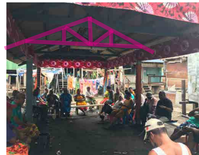
Figure 49: Gable Roof truss with bracing. Location: Ontong Java settlement (Photo credit: John Clemo)
