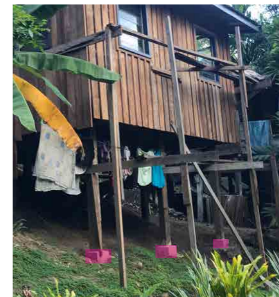
Figure 38: Photo of a house built on reinforced concrete pad footing with timber post. Location: Aekafo-Feraladoa settlement (Photo credit: John Clemo)
