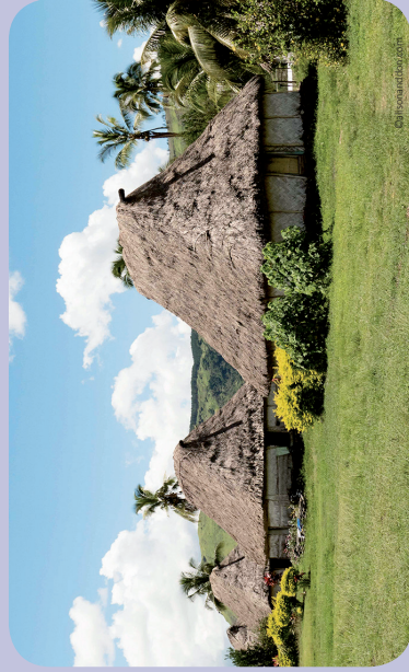
Eaves are narrow in traditional bure houses in order to minimise roof tearing caused by winds
