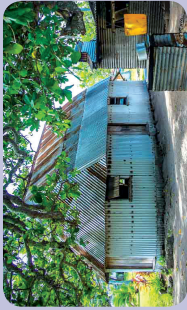
Rounded corners are found in either traditional and new built houses. This house is built with CI sheets
