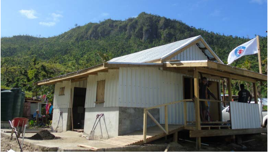
Core shelter built after TC Winston (Fiji Red Cross/IFRC)
