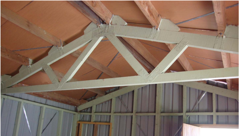
This house survived unscathed from TC Winston, when nearly all else around it was destroyed. Note strapping on every joint, diagonal bracing on the wall and roof panels and metal plates on the truss timbers. (Source Habitat for Humanity)
