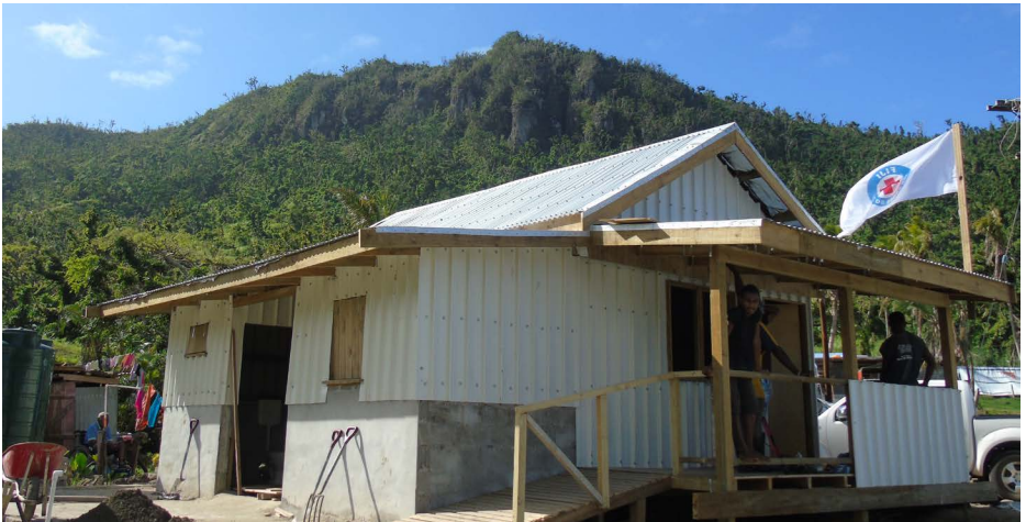
This house was built after TC Winston with Build Back Safer principles. (Source Fiji Red Cross Society/IFRC).
