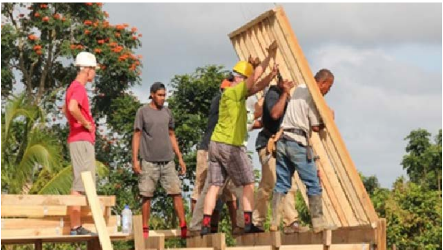
Habitat for Humanity Fiji team at work to build shelters and train people to build back safer. (Contact hfhfiji@habitatfiji.org.fj Ph: 3312012)
