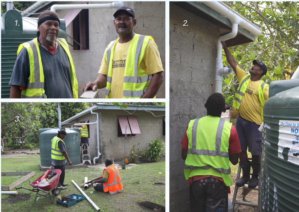
Images: 1. Brothers (L) Bill and Timoci Ravovou. 2 & 3. Installation of a First Flush Device. © Habitat for Humanity Fiji
